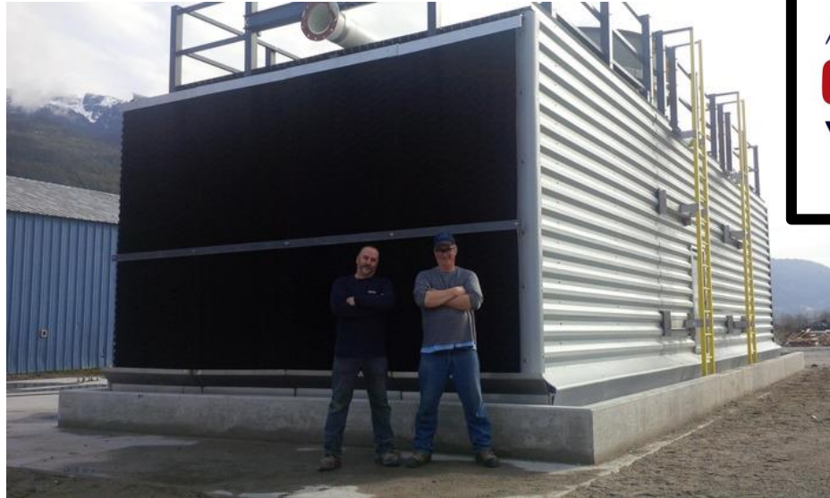
Squamish demo plant site construction
